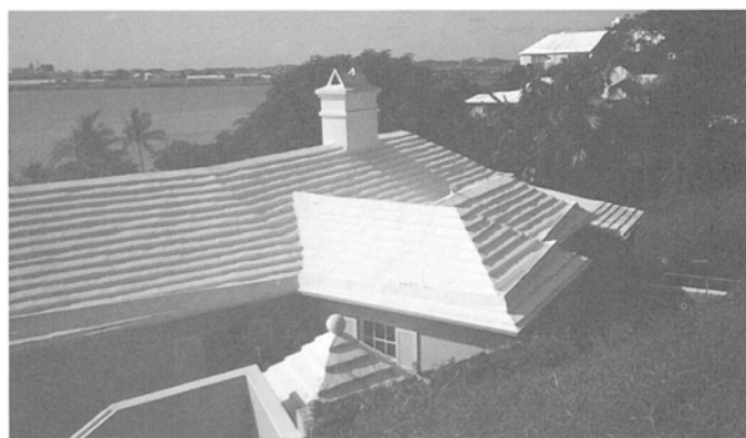
Fig. 6. Roofs of Bermuda dwellings are painted white, principally as a means of maintaining water collection, and have the effect of dramatically reducing solar heat gain.
